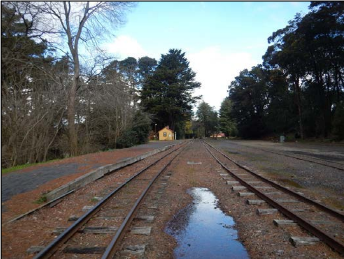
Plate 87 Railway tracks approaching Gembrook Station, facing south-east (L. Tepper 4/9/17)
