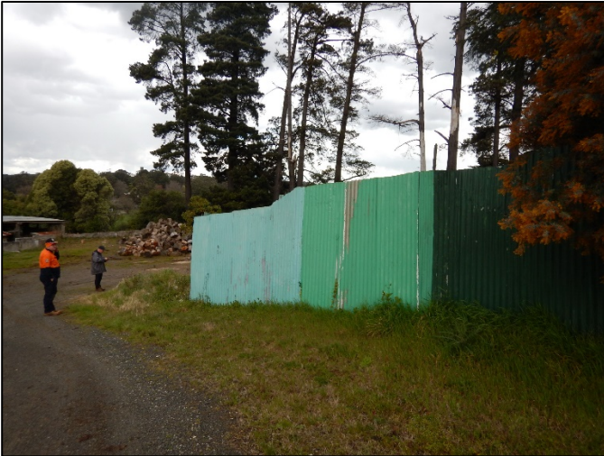
Plate 82 Corrugated metal fence and gravel driveway, facing south (L. Tepper 4/9/17)
