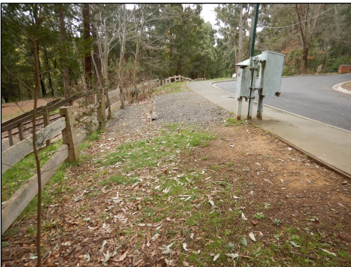
Plate 67 Services located within the survey unit, facing north (L. Tepper 4/9/17)
