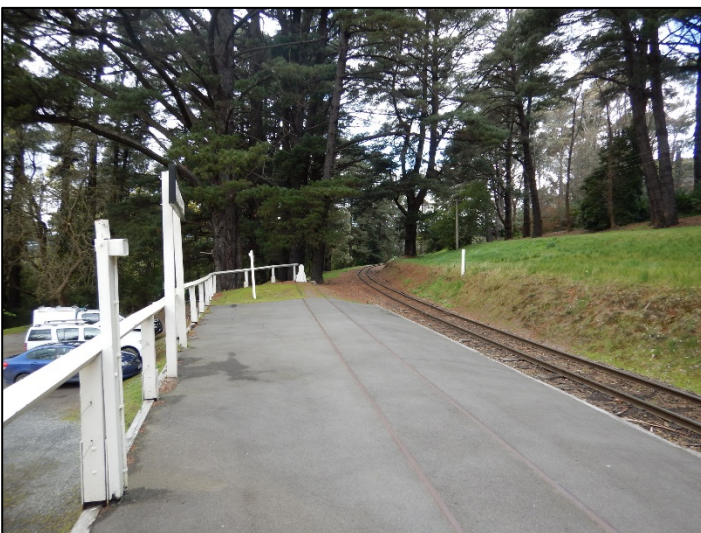
Plate 56 Siding and railway track facing east, showing stepped cutting (L. Tepper 4/9/17)
