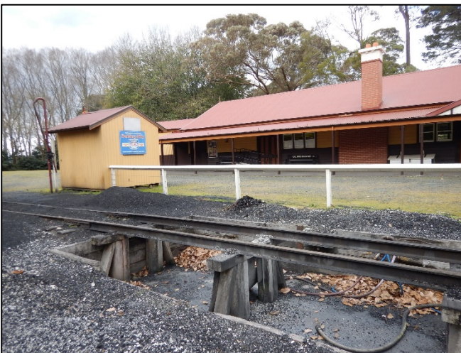
Plate 94 Underground inspection pit and station buildings in the south of the survey unit, facing east (L. Tepper 4/9/17)
