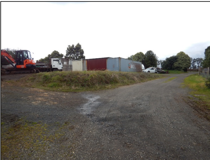
Plate 80 Gravel driveway, equipment and storage containers facing north (L. Tepper 4/9/17)
