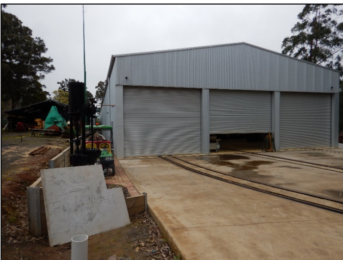
Plate 35 Large workshop on concrete pad in the south of the survey unit, facing west (L. Tepper 4/9/17)
