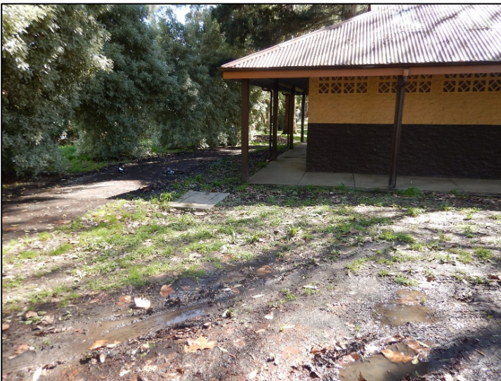
Plate 46 Toilet block and sewerage system, facing north-west (L. Tepper 4/9/17)
