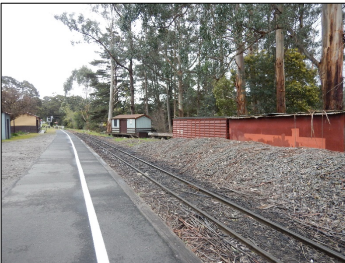
Plate 34 Railway tracks, ballast and associated buildings, facing west (L. Tepper 4/9/17)
