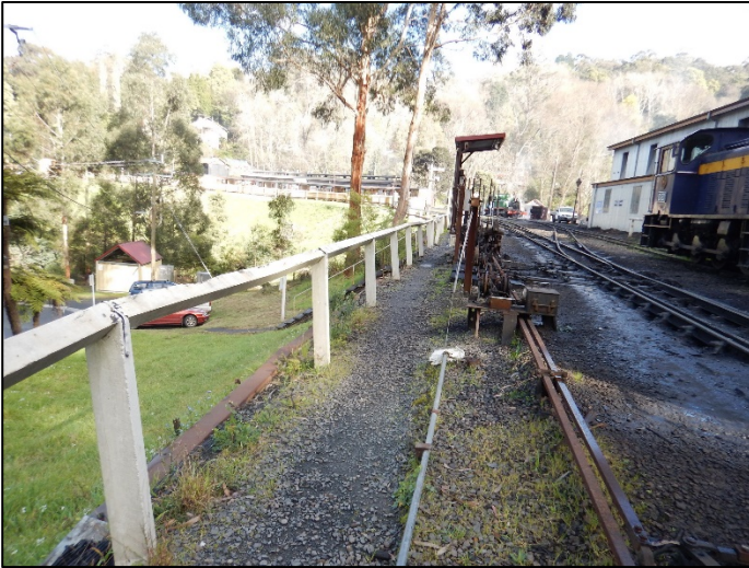
Plate 25 Area of cut and fill below ballast and railway tracks, facing west (L. Tepper 4/9/17)
