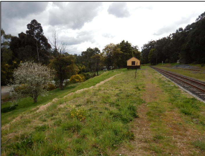
Plate 75 Station platform facing north, showing grass coverage (L. Tepper 4/9/17)
