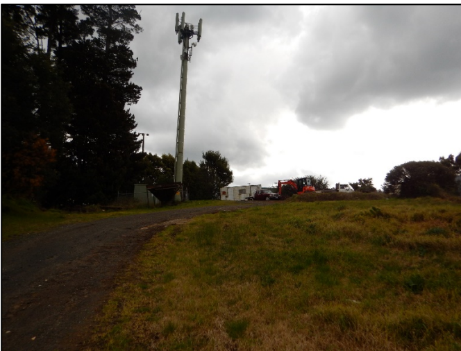
Plate 83 Telecommunications tower within the south-west extent of the survey unit, facing north-west (L. Tepper 4/9/17)
