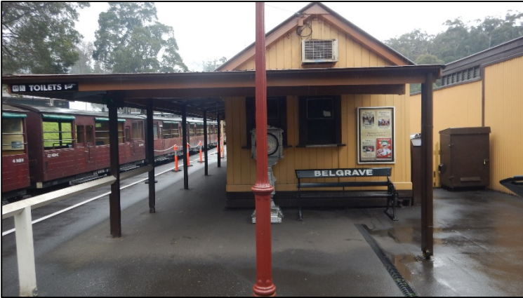
Plate 19 Belgrave Station platform, facing north (L. Tepper 4/9/17)
