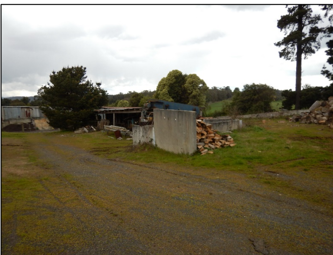
Plate 81 Concrete wall and stockpiles of timber, facing south-east (L. Tepper 4/9/17)
