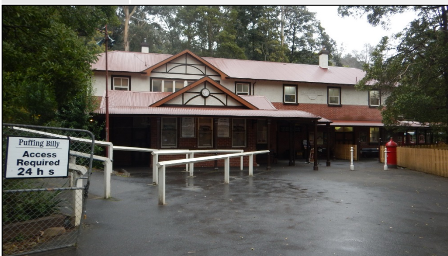
Plate 18 Belgrave Station building, facing west (L. Tepper 4/9/17)
