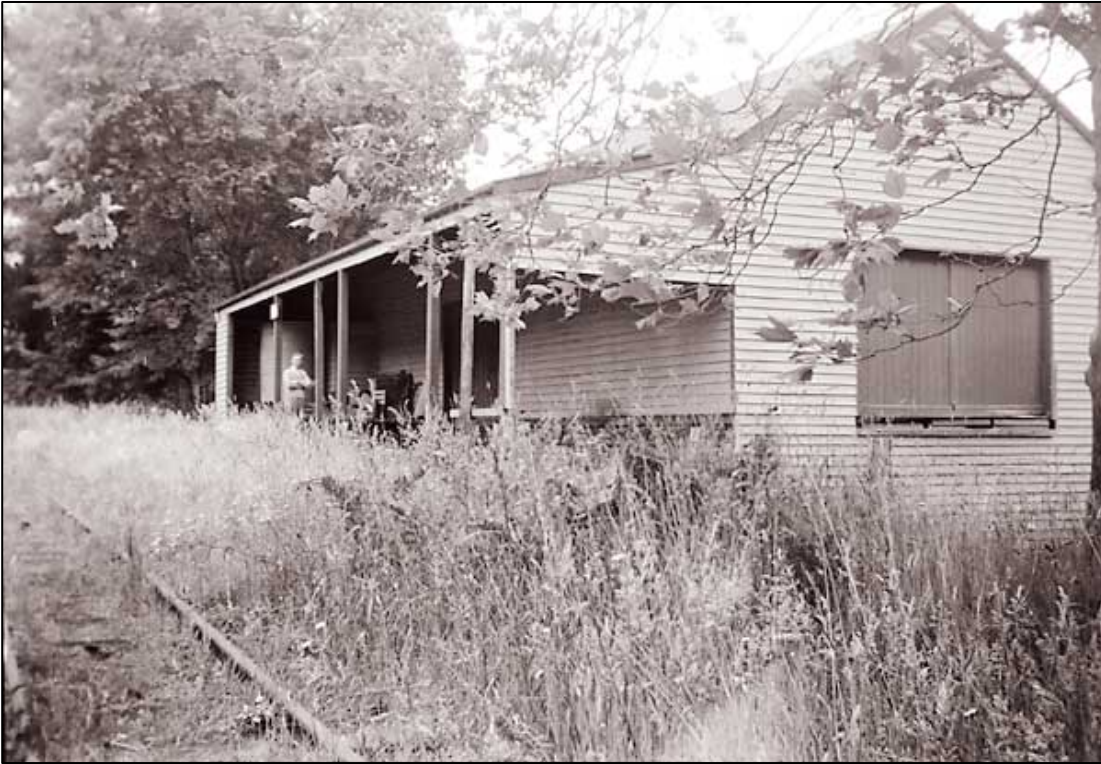
Plate 12 Nobelius packing shed and siding c.1955 (Photo Frank Stamford)
