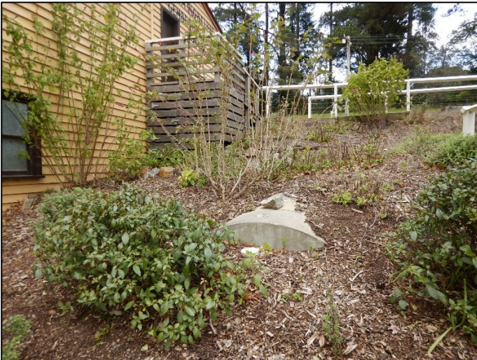
Plate 61 Services within garden bed, facing south (L. Tepper 4/9/17)
