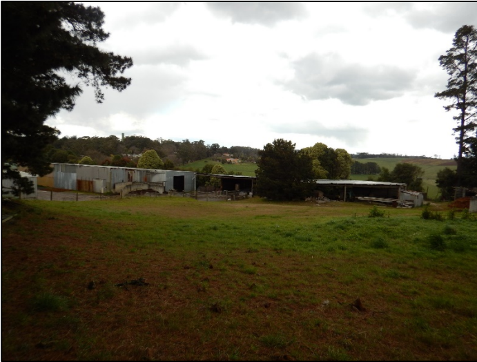
Plate 79 Gembrook Workshop site facing south-east showing sheds and equipment (L. Tepper 4/9/17)
