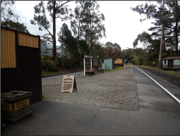
Plate 33 Platform and station buildings, facing west (L. Tepper 5/9/17)
