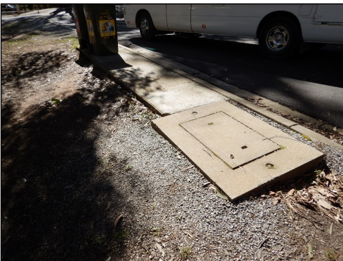
Plate 68 Drain located within survey unit (L. Tepper 4/9/17)
