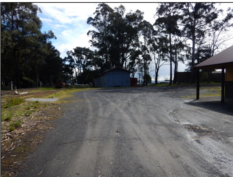
Plate 44 Gravel driveway leading from Puffing Billy Place to the workshops, facing south (L. Tepper 4/9/17)
