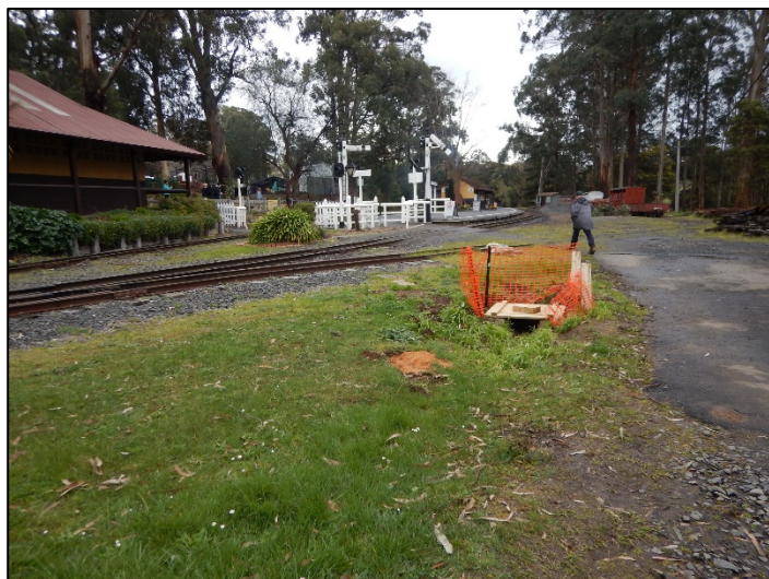
Plate 32 Facing towards Menzies Creek Station and toilet block, facing west (L. Tepper 4/9/17)
