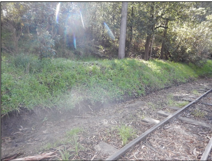
Plate 29 Area of proposed siding, facing north-east (L. Tepper 4/9/17)
